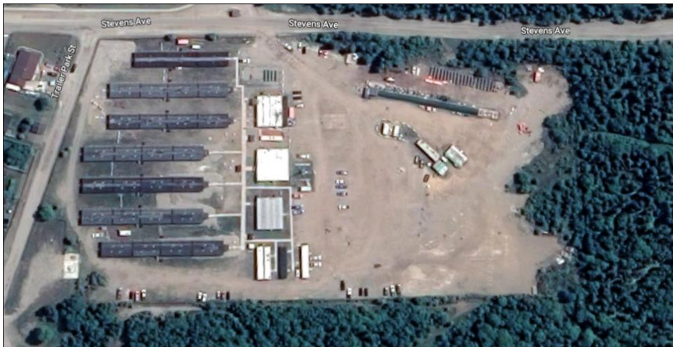
Figure 18-17: Marathon Construction Camp
